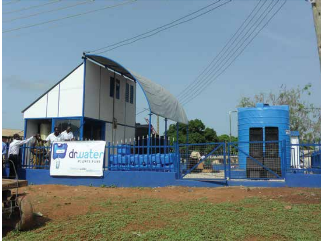
Water treatment plants like this one in the Greater Accra region are manufactured as kits that can be easily assembled and maintained by local workers.
