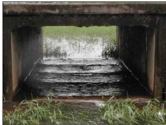
Figure 1. Fish-friendly designs for high water velocity barriers (example of a culvert design creating controlled water velocities and increased depth to facilitate fish passage in Queensland, Australia)
