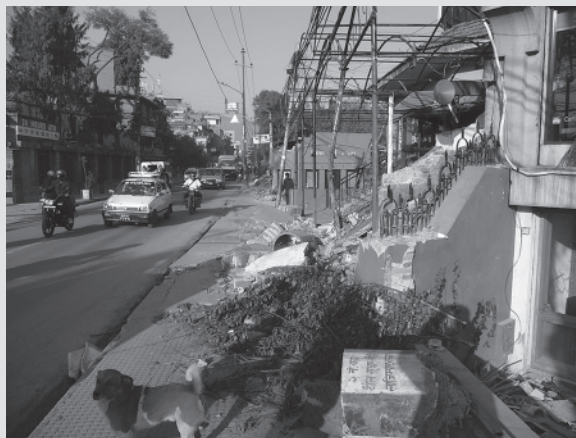
Figure B6.4.1 Demolished Buildings to Enforce Right of Way
