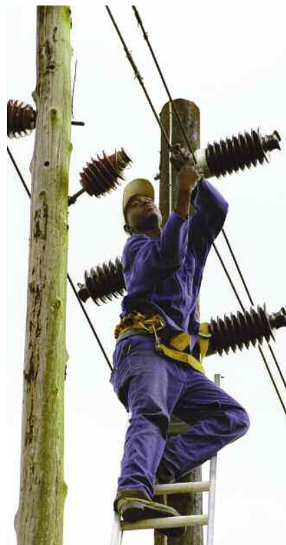
Working on electrical power lines outside the town of Macia, Mozambique.
